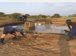
7. BACKFILLING AND COMPACTION
