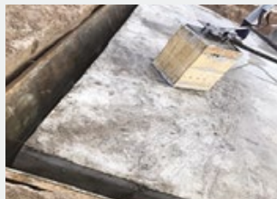
6. REMOVAL OF FORMWORK
