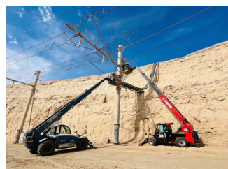
Installation Work in progress on Trolley Line#05
