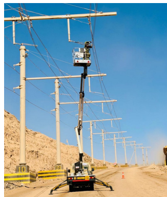
Trolley Line#04 Maintenance with Cherry Picker
