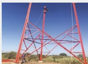
8. RIGGING OF TOWER
