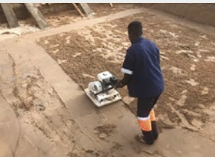
1. COMPACTION OF BASE FOUNDATION EXCAVATION
