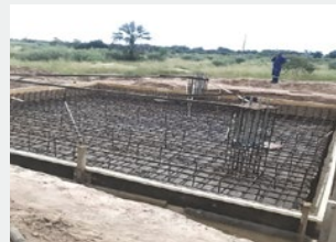
3. REINFORCED STEEL FIXING FOR BASE FOUNDATION
