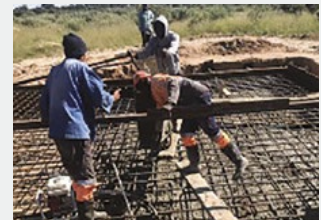
4. CASTING OF CONCRETE FOR BASE FOUNDATION
